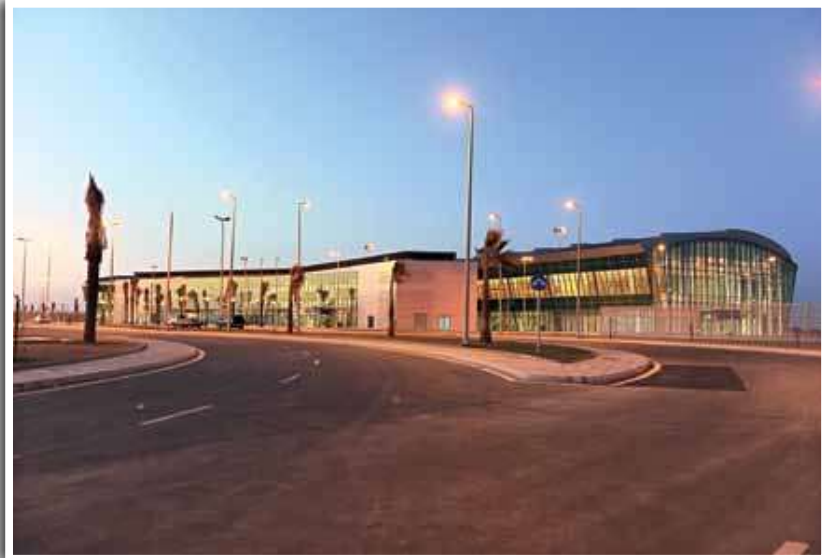
Prince Sultan bin Abdulaziz airport (PSAA) in Tabuk
